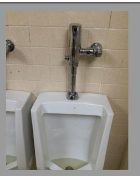
FYI, you can't just retrofit a new 0.125 gpf flush valve on an old 1.5 gpf urinal and expect it to work. It won't. The result: Diluted urine sitting in the bottom of all the urinals.
