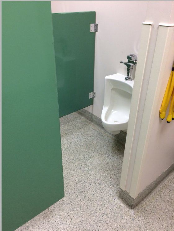
Seriously? Who designed this ADA compliant toilet room???
