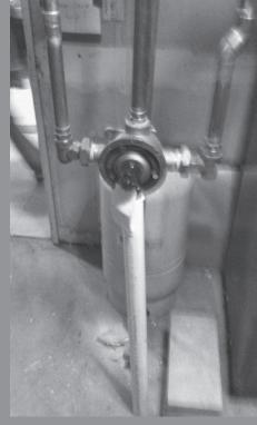
Left: You are in luck this month. I have a second plumbing installation photo for you. This was a Southeastern MA area mixing valve installation. Apparently the plumber decided the best way to support the building's new mixing valve was to cut a 30" section of PVC pipe and use it to prop up the mixing valve off the floor. Brilliant!
